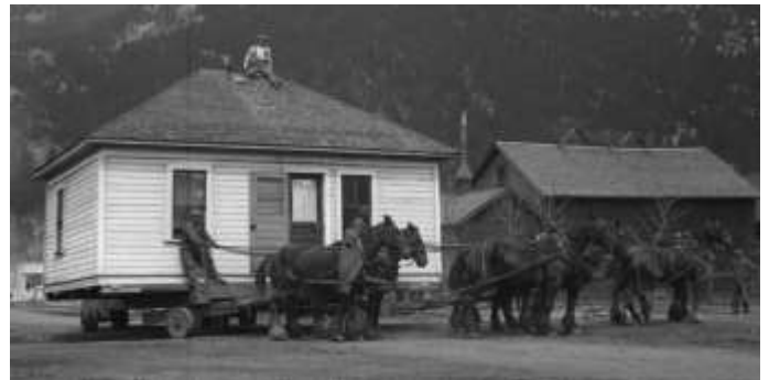
Turning a corner, Blairmore, 1935. In the background is the Gushul Studio, a building moved from Lille.
