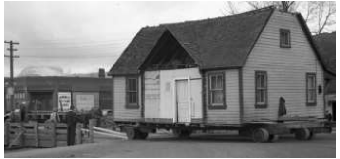
A Hillcrest house crossing the Lyon Creek bridge, 1945. The roof spine has been trimmed to clear obstacles. The story goes that the lady of the house rode inside to keep an eye on her furniture and dishes during the move, and had to spend the night when the house movers stopped at the Frank Hotel to celebrate the end of the war!
