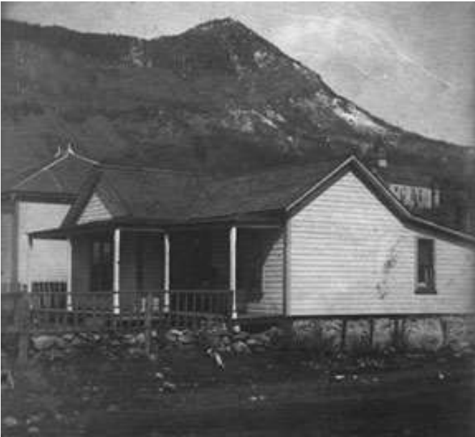
Naylor residence, 1910, in Frank on the northwest corner of Ninth and Dominion, today's 15045 - 21 st Avenue. Built in 1906, the house was gone by 1919. Crowsnest Museum and Archives, Kerr 0566a
