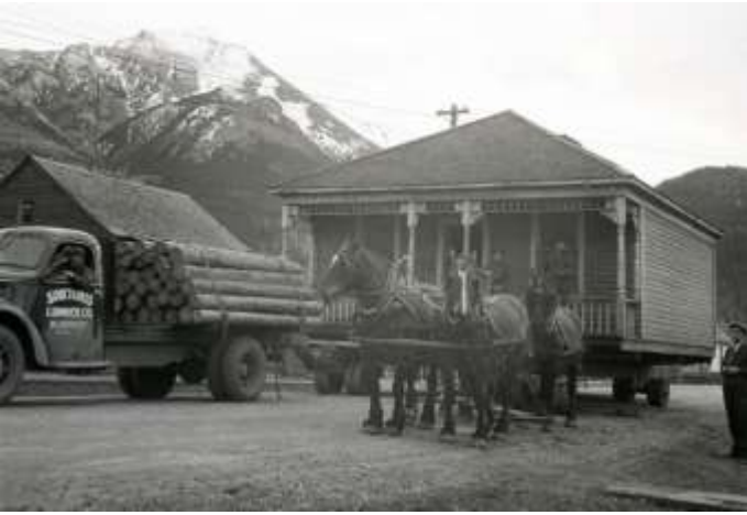
A house heading north in the Pelletier Addition (south Blairmore), horse/truck combo, about 1940.
