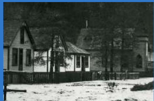
W. T. Young residence (centre) during the 1923 flood. All four buildings in the photo still exist. Photo: Crowsnest Museum and Archives
