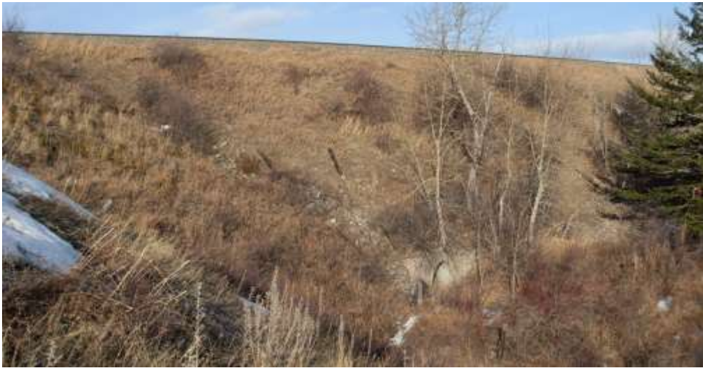
The earth-filled coulee near Burmis today. It may be the same coulee as that shown in the previous photograph, but here viewed from the other (south) side. The concrete culvert portal can be seen at the base of the earth-fill.
