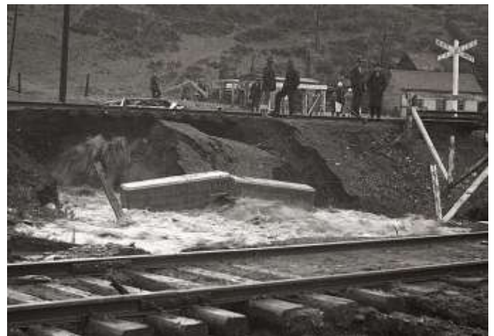
The 1910 Nez Perce Creek culvert during the 1923 flood. Photo: Crowsnest Museum and Archives, 6044 Gush Neg
