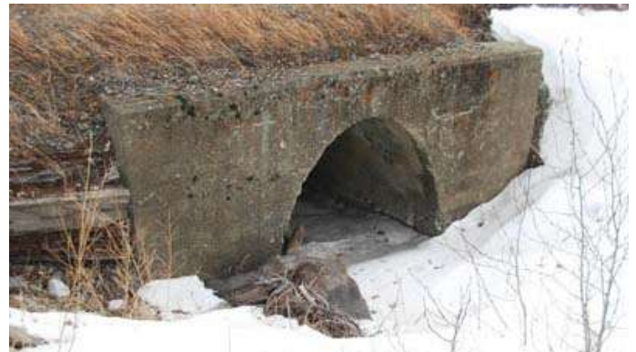
The 1923 Nez Perce Creek replacement culvert today. Photo: Ian McKenzie
