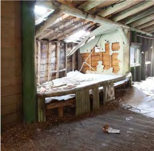
Left: the stage, with roof holes and drifted snow
