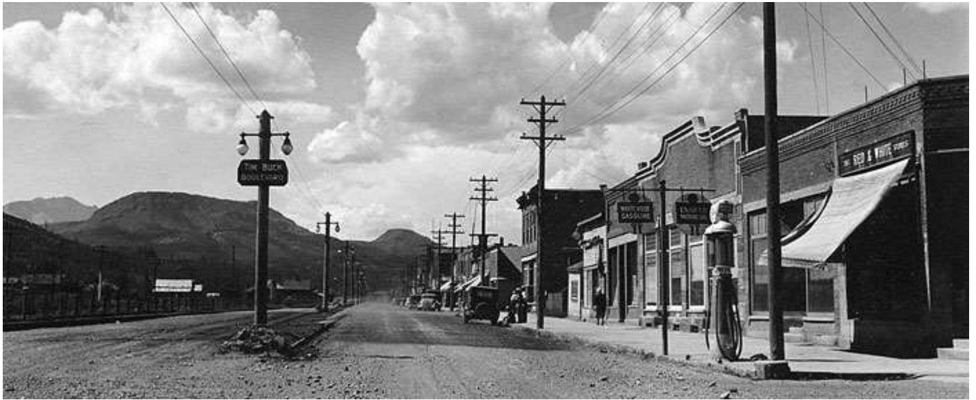
Tim Buck Blvd, sprinklers suppressing street dust.
