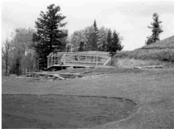
New clubhouse under construction – c. 1955
