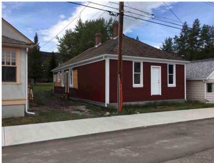
Restoration of Building as of June 4, 2017 (Fred Bradley Photo)
