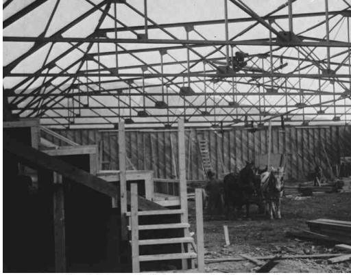
Crystal Arena in Coleman under Construction
