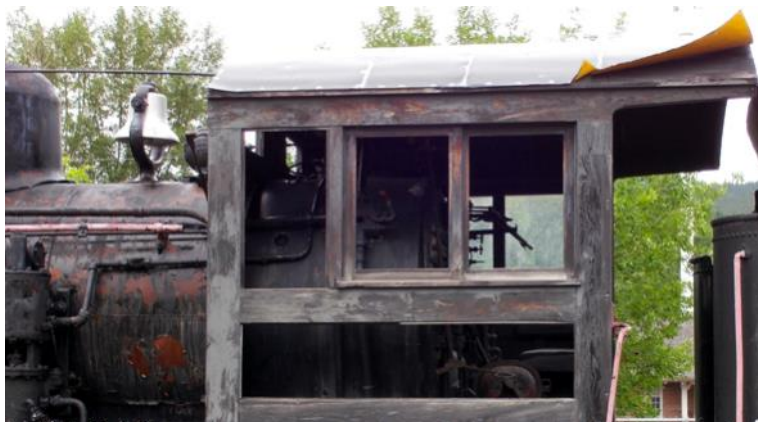
Old Maude., Blairmore Main Street. Note the peeling roof and rust. Photo by C. Allum 2012.
