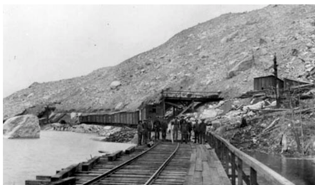
Rebuilding railway line. Glenbow Archives. NA-672-3
